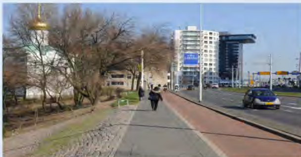
70 year protection Inside Rotterdam, levees are incorporated into the urban fabric as inhabitable public spaces.
