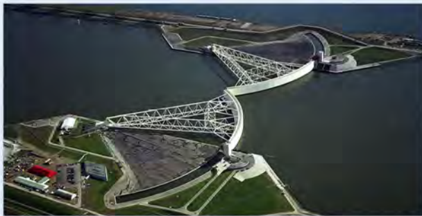
100 year protection The Maeslant Barrier, a Delta Works project outside Rotterdam, is the city's first line of defense, closing to stop storm surges from the North Sea.
