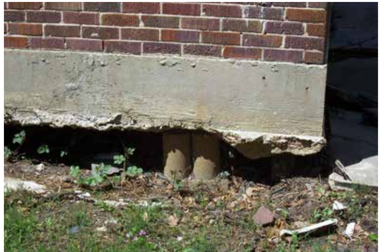
Exposed foundation and wood pile decay risk due to subsidence
