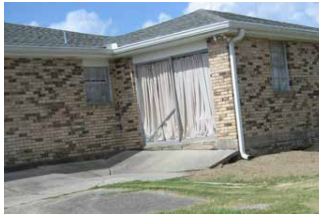
Subsidence results are evident in depressed driveways and exposed foundations in Village de l'Est, New Orleans East
