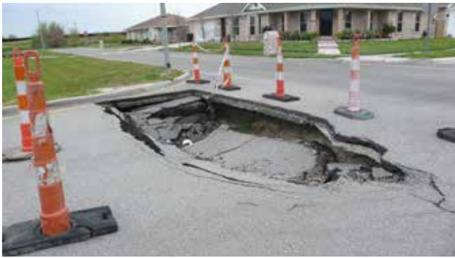
Severe street damage due to subsidence in St. Bernard Parish
