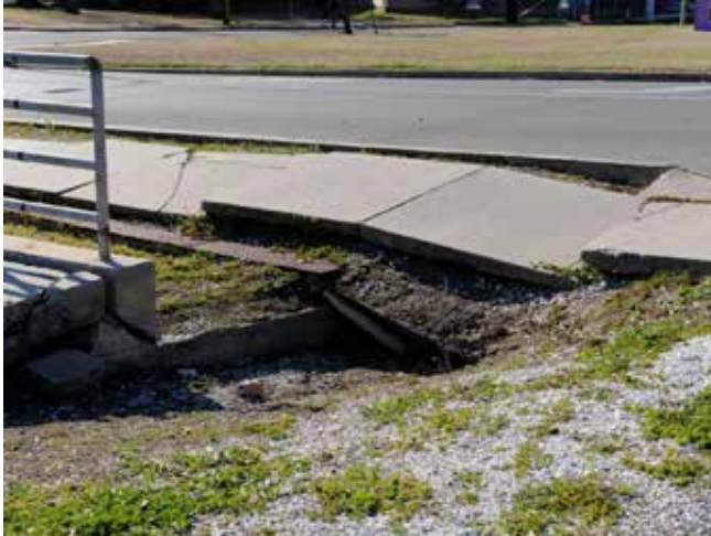
Buckled sidewalk due to subsidence
