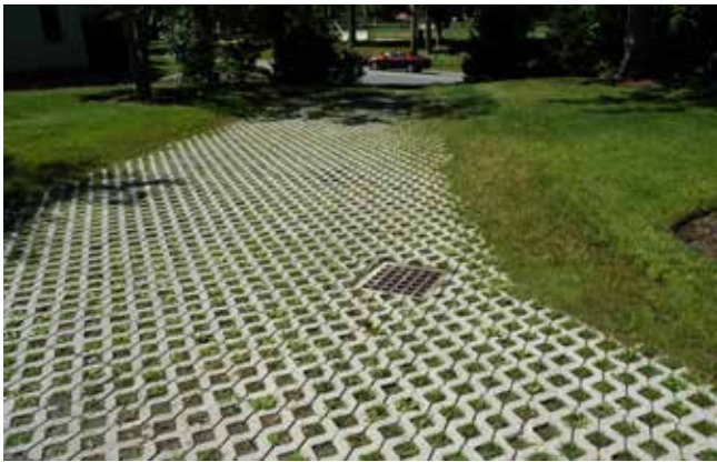
Reduce impervious surfaces by installing stormwater management best practices including green roofs and pervious paving
