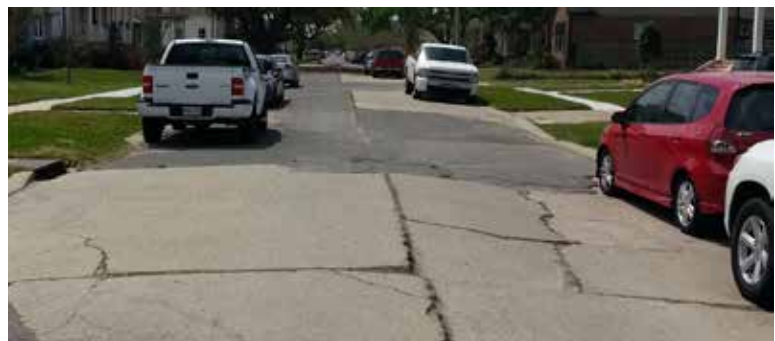
Broken streets common in the Lakeview area (pictured here) and elsewhere due to differential ground settlement
